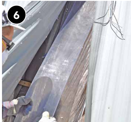
6 Insert batt into cavity, sliding under top belt rail to top of cavity, and pull the stuffing tool back out to allow batt to fill in space.
