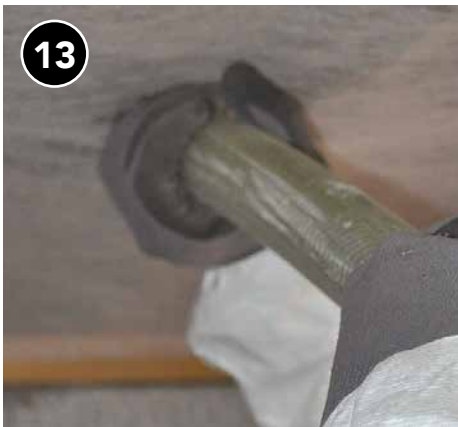
13 Loose fill netting to required density.
