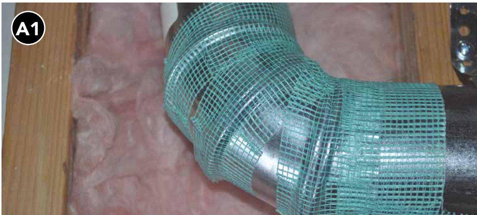
Apply fiberglass mesh tape over all gaps, seams, joints, etc.
