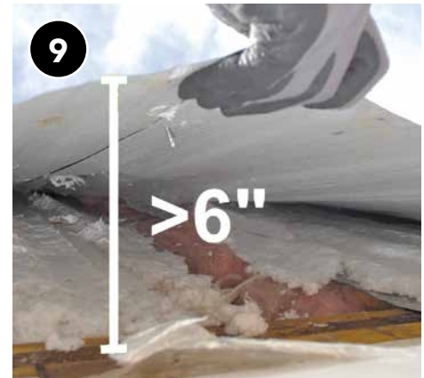
9 Work down the edge of the roof until entire cavity is full.
