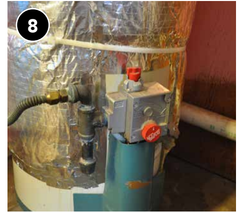
Secure seams with tie strap, wire, or twine and minimal compression.
