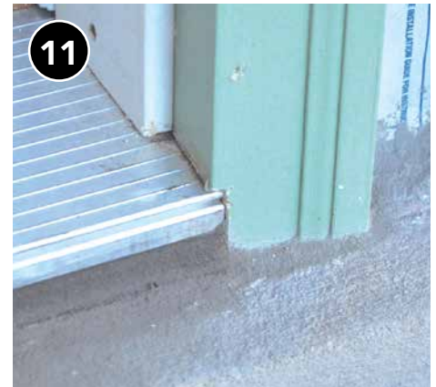
Seal along threshold, ensuring water will flow away from door.
