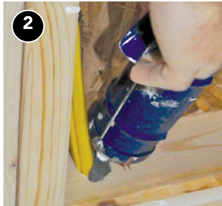
2 For smaller gaps, caulk is enough to seal the hole.
