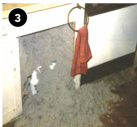
Confirm the wall integrity can withstand the air pressure of blown insulation and make sure all holes are repaired to prevent insulation blowouts.
