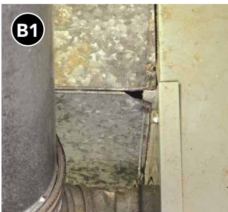
Small holes and penetrations require one additional step.
