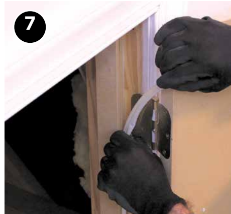
For vertical accesses, run weatherstripping or closed cell foam tape to air seal at these doorways too. Hold vertical accesses closed with latch if necessary.
