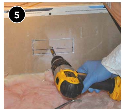
Patch all access holes in backing material. Use access hole plugs when a rigid material is used or seal slits in house wrap material with a high quality tape.
