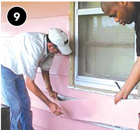
Carefully reinstall any removed siding.
