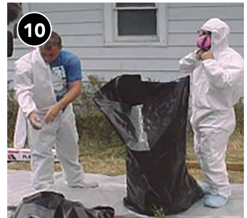
10 After stepping on a tack pad and using a HEPA vacuum to clean residual dust; remove PPE outside, taking care to avoid contact with contaminated surfaces of the suit, gloves, etc. Dispose of PPE in a plastic waste bag.
