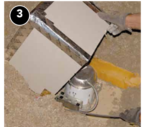
3 Premade boxes can make installation easier when installation site is clear of framing members.
