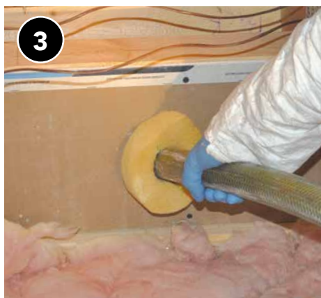
Blow insulation into cavities to meet dense-pack standards.
