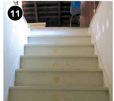
Plug access holes for blown insulation.
