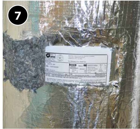
Cut flaps at access plates, tape them shut and then label from the exterior.
