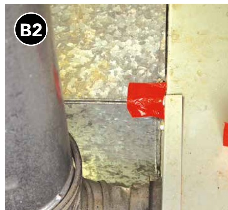
Apply temporary UL-listed or mesh tape as a backer to hold mastic.
