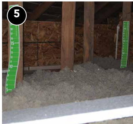
5 Insulation depth rulers installed, 1 per 300 square feet.
