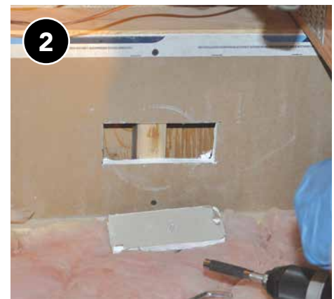
Cut holes in rigid backing material or cut small slits in house wrap material to allow access to each cavity.
