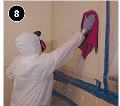
8 Wipe down surfaces and vacuum work area, taking special care and attention with cracks and crevices where dust and debris might collect.
