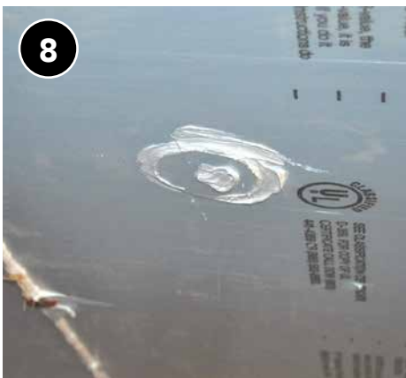
8 Seal around plug to keep it secure and air tight.
