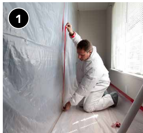
Protect the floor below the work area and use containment enclosures to prevent the spread of dust and debris.
