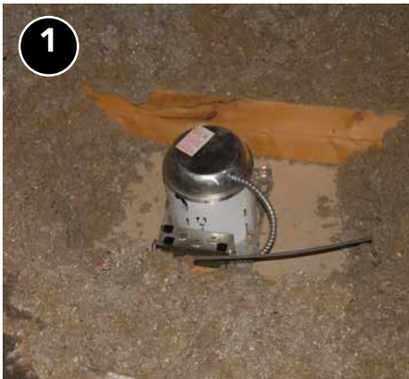
1 Clear any debris and insulation from around non-IC rated can light.
