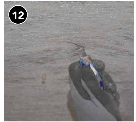
12 Cut access hole for fill tube.
