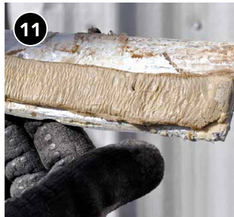
11 Replace butyl tape on J channel.
