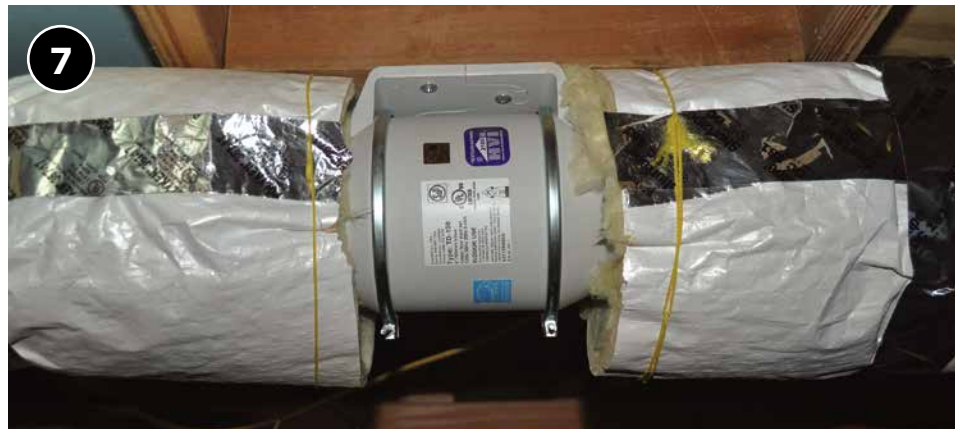
7 If duct run must exceed 35 feet, install booster fan.
