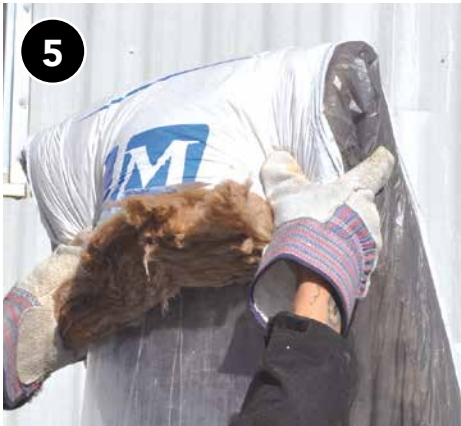
5 Fold the batt over the insulation stuffing tool.
