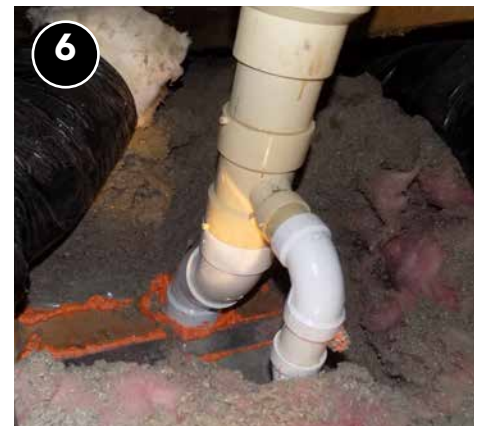
6 Other penetrations such as plumbing vents can be sealed using foam or caulk with backer rod as described in step 4.
