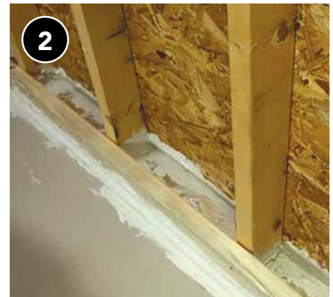
Ensure balloon-framed walls are blocked at top and bottom to prevent insulation from unintentionally blowing into the attic or basement.
