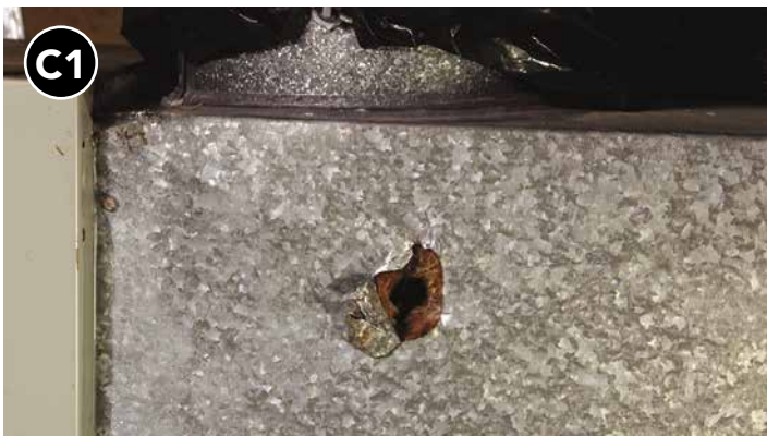
Larger holes require a different process.
