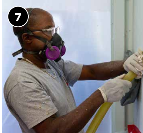
Dense pack stairway walls.
