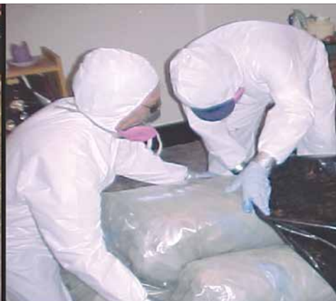
9 Carefully roll up disposable physical barriers, folding the dirty side inward and dispose of any plastic sheeting or other disposable materials in the work area.
