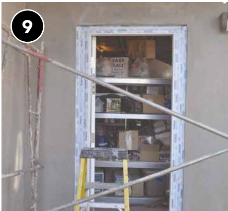
Seal rough opening to prevent both air and water intrusion.
