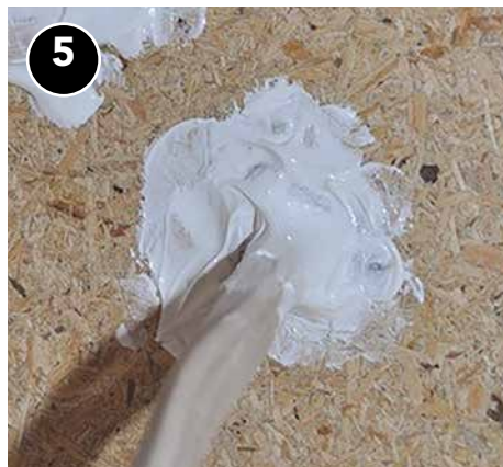
5 Seal to cover entire opening, including all backer rod.
