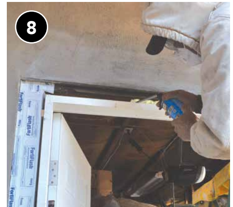
Insulate gaps between door jamb and frame.
