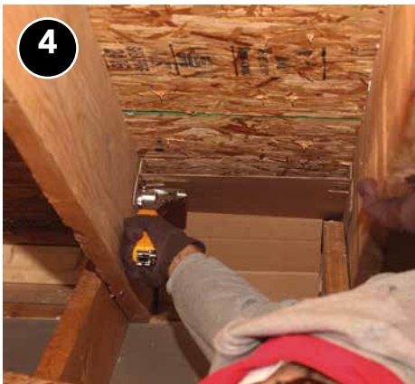
4 Install baffles, if needed. Ensure 1–2 inches of space between the baffle and roof decking for airflow.
