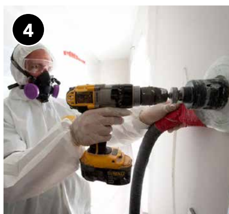
Drill insulation access holes as needed to ensure complete coverage of all uninsulated wall cavities.
