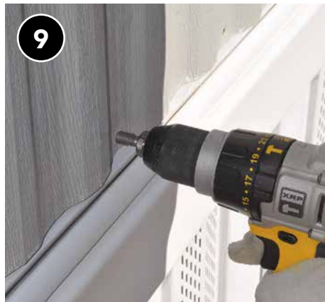
9 Reattach mechanical fasteners.
