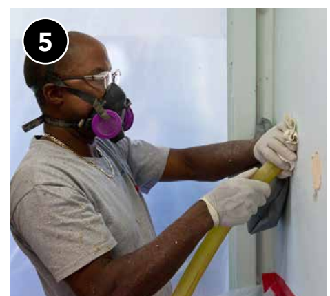
Fill cavities completely and to the proper density.
