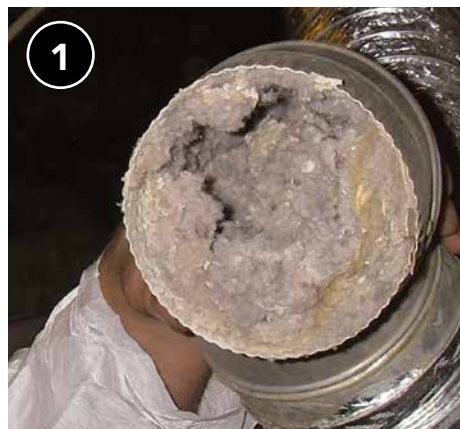
Keep duct run as short and straight as possible to prevent backup of lint.
