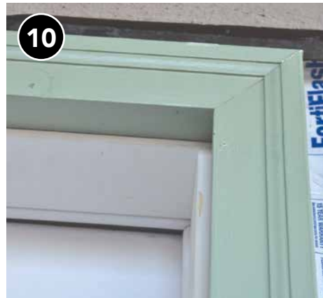
Reinstall existing trim or secure the trim supplied with the pre-hung door unit.
