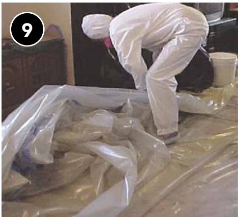
9 Carefully roll up disposable physical barriers, folding the dirty side inward and dispose of any plastic sheeting or other disposable materials in the work area.
