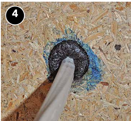
4 Inserting backer rod provides infill to support the sealant.
