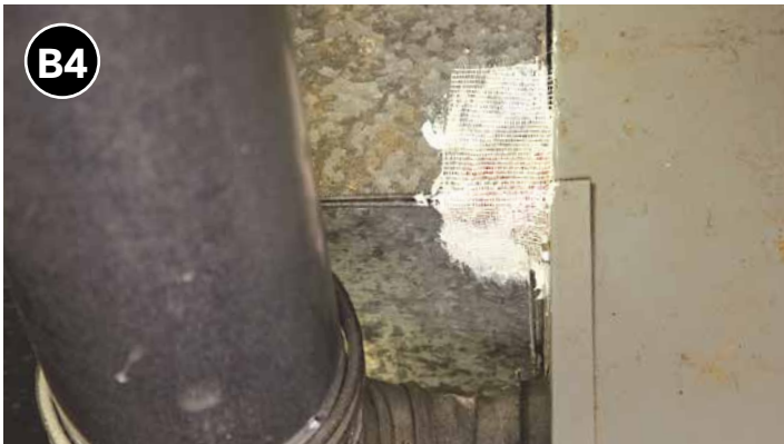
Push fiberglass mesh into the mastic.
