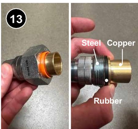
Install dielectric unions when connecting copper to galvanized steel piping in accordance with IRC and manufacturer specifications. **7.0302.3j.**
