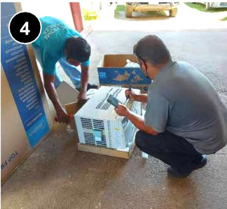
Remove the new AC unit from its packaging and ensure the physical size will fit in the current hole without blocking vents. **5.0301.1a.**
