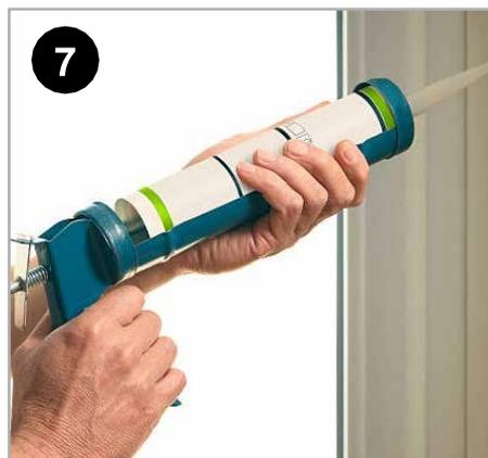
Before installing through-wall unit, seal all adjacent framing and provide a sealed and sleeved opening. After installation, seal the perimeter with suitable materials. **5.0301.1e.**
