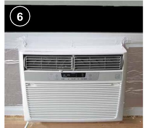
Mount the unit, leveling from left to right, keeping the unit's mounting surface flush with the inner surface of the mounting bracket, frame, or window as per manufacturer instructions. Ensure the unit's condensate drain is at the lowest possible point, sloped away from the unit and the building.
