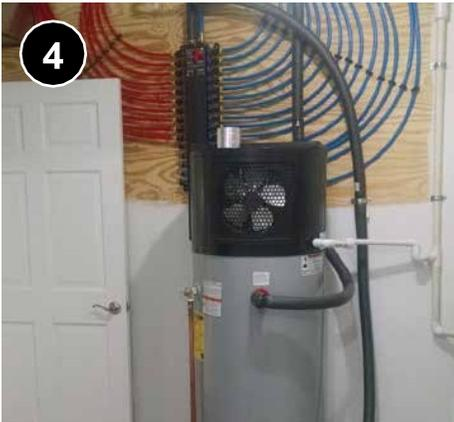
4 Ensure the room meets requirements for the unit. Is there enough volume and clearance for airflow around the unit? Are the ceilings high enough? Is there adequate space to allow maintenance of the heat pump components, including removal and cleaning of the air filter? Ensure the unit will not blow directly on an indoor thermostat or occupants. [7.0302.3c.](#)
