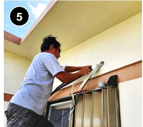
Drill hole(s) for control wires and the condensate and refrigerant lines (preferably one, but multiple if necessary).
