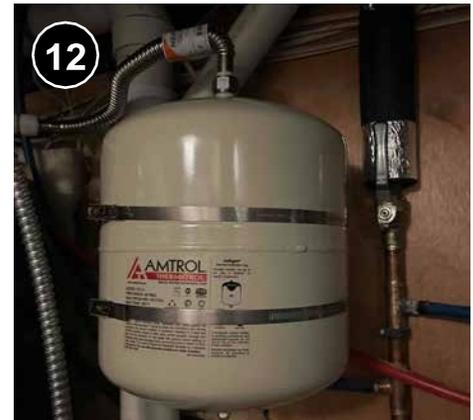
Support the expansion tank so that it does not move or sag using rigid support material that is able to support twice its weight when filled with water. [7.0303.5d.](#)
