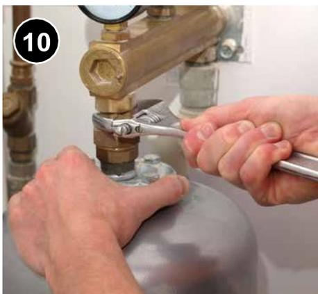
If the cold water supplying the HPWH passes through a check valve, **pressure reducing valve (PRV)**, or backflow preventer, install an expansion tank on the cold-water supply line at a point that is downstream of all those valves. Size the expansion tank in accordance with manufacturer specifications and applicable code. **7.0302.3i.**
