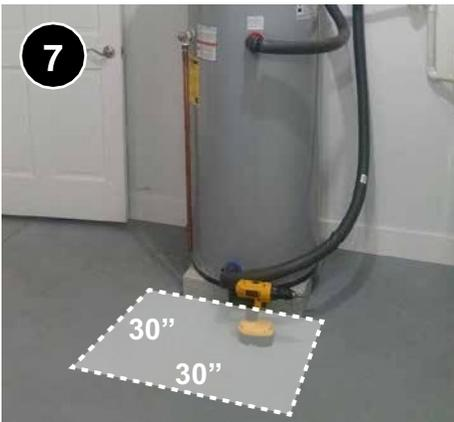
7 Double check clearance in front of the unit's control side to allow at least 30" x 30" to allow for inspection, maintenance, and replacement of components. [7.0302.3e.](#)
