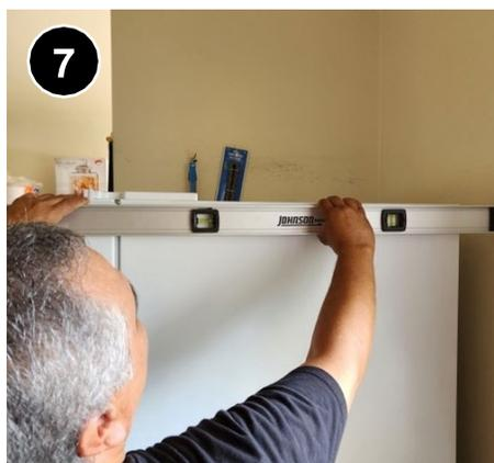
Now check for level front to back, again using the frame of the refrigerator. You will want the unit to lean slightly to the rear, so the door gently closes on its own. Adjust the feet if necessary.
