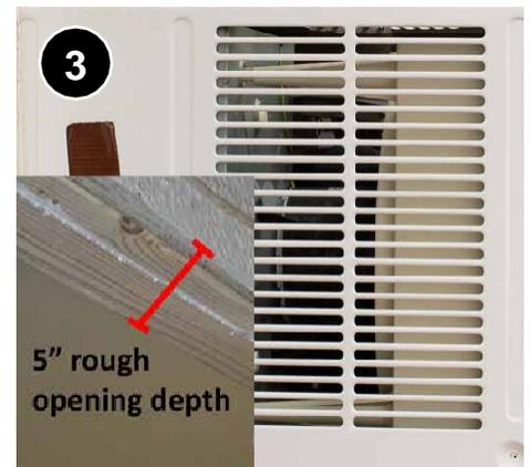
Measure the thickness from inside wall surface to the outside covering of the home. The wall thickness must not exceed the non-vented portion of the AC unit mounting assembly or unit itself (i.e., when installed, AC vents must not be blocked in any way).
