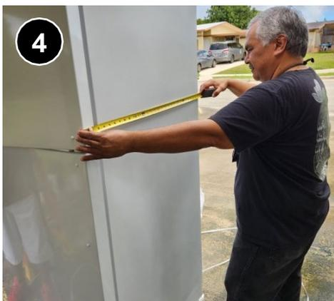
Clean the floor area where the new refrigerator will be placed. Measure to ensure the refrigerator will not block access to light switches, cabinets, etc., and will fit through the smallest opening between the outside and the installation location. **7.0101.1b.**
