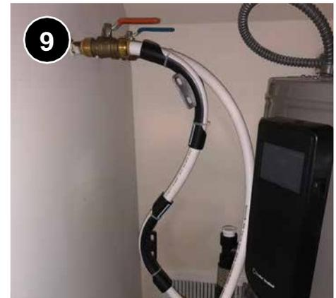
9 If not already present, install separate water cut-off valves for both hot- and cold-water lines. [7.0302.3h.](#)
