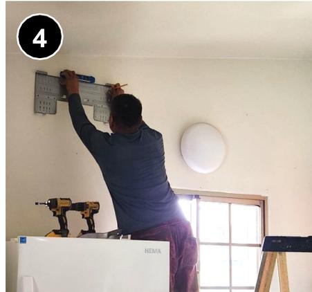
Securely fasten the mounting bracket to the wall, level, using appropriate anchors. The bracket must be installed following manufacturer specifications and in accordance with applicable building codes. [5.0108.3g.](#)
