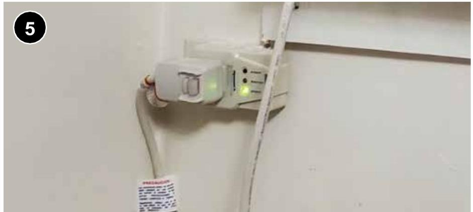
Ensure the supplied electrical cord is of sufficient length to reach the nearest outlet that meets the requirements of **NFPA 70 Article 422** (Maximum breaker size for the circuit matches or exceeds the breaker marking on the appliance). It is not allowable to plug the unit into an extension cord. Therefore, if the cord does not reach, proceed with one of the following options, based on the recommendation of the auditor and available funds:
