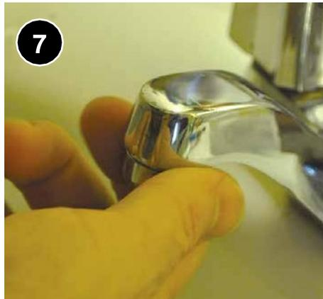
Carefully install new aerator without over tightening. Ensure rubber washers are in place and take care not to cross-thread.
