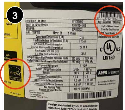
Select a new HPWH that is ENERGY STAR® certified, equivalent, or better and fits in the installation space with appropriate clearances and provides sufficient hot water for the home and occupants. [7.0302.3b.](#)
