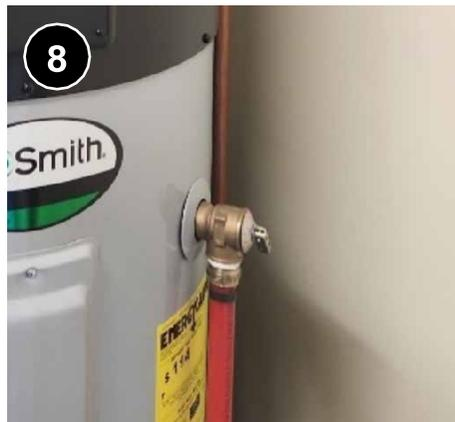
8 Install a Temperature and Pressure (T&P) relief valve per IRC and manufacturer specifications. Pipe the valve to within 6" of the floor or drain pan, or directly to the outdoors in an observable location. Piping material must meet IRC requirements. [7.0302.3f.](#)
