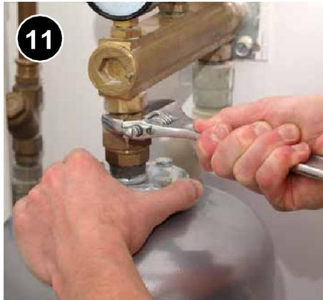
If the cold-water supply passes through a check valve, pressure reducing valve (PRV), or backflow preventer, install an expansion tank on the cold-water supply line at a point that is downstream of all those valves. Size the expansion tank in accordance with manufacturer specifications and applicable code. [7.0302.6l.](#)
