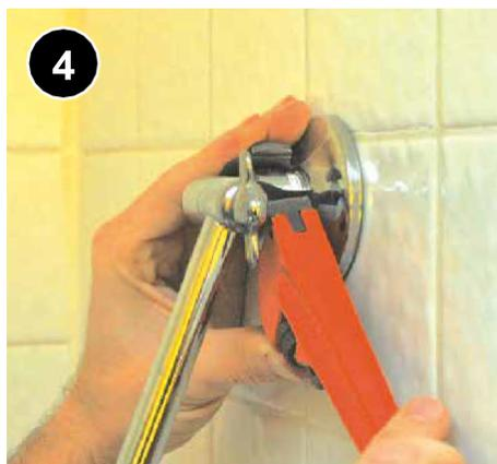
4 Then use pipe wrench or channel locks to loosen connection at shower arm.
