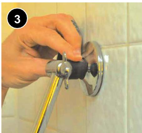
3 If old showerhead does not have flat sides at connection, wrap with buffer material, such as a piece of rubber.
