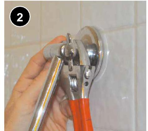
2 Carefully remove old showerhead with adjustable wrench, taking care not to loosen shower arm.
