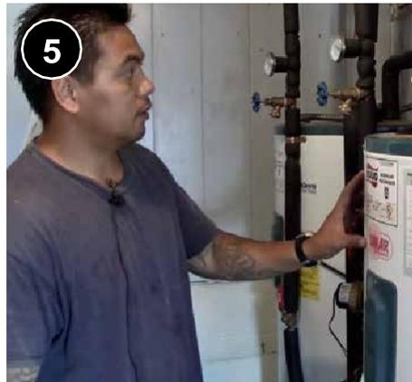
Select a storage tank/backup water heater that is ENERGY STAR® certified, equivalent, or better; fits in the installation space with required clearances; provides sufficient hot water for the home and occupants; and is insulated to R-12.5 or greater. [7.0302.6b](#).
