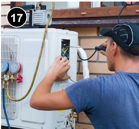
At this point, an electrician will need to make the final electrical connections and a trained technician will purge the system with nitrogen to check for leaks, remove nitrogen and moisture from the system and open the outdoor valves to release refrigerant into the system.
