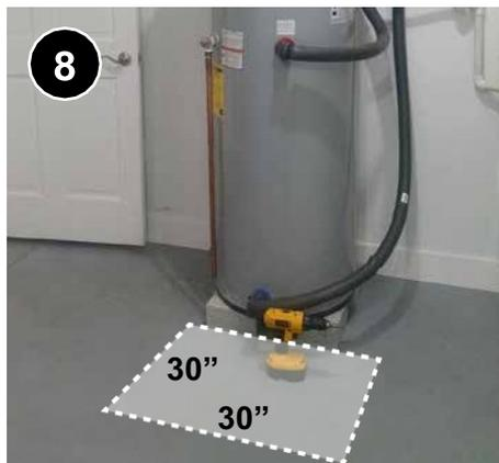
Double check clearance in front of the storage tank to allow for inspection, maintenance, and replacement of components (including replacement of the anode rod). [7.0302.6e](#).
