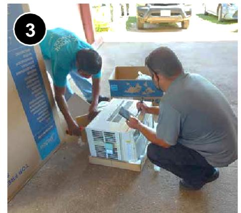
Double check the name plate of the new AC unit to ensure the new unit meets the requirements of the program. The new unit must match existing voltage and have a CEER of 12 or higher of the same or lesser capacity (when compared to the unit it is replacing). **5.0301.1b.**
