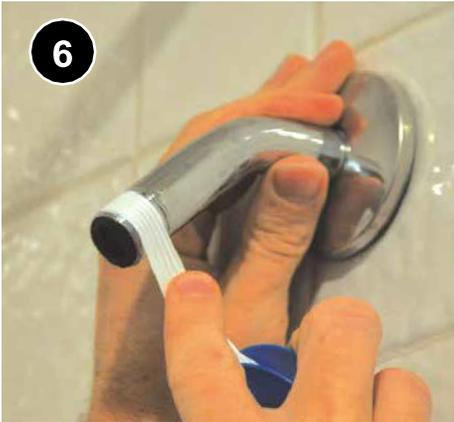
6 Wrap new thread tape around threads. [7.0201.1c](#)
