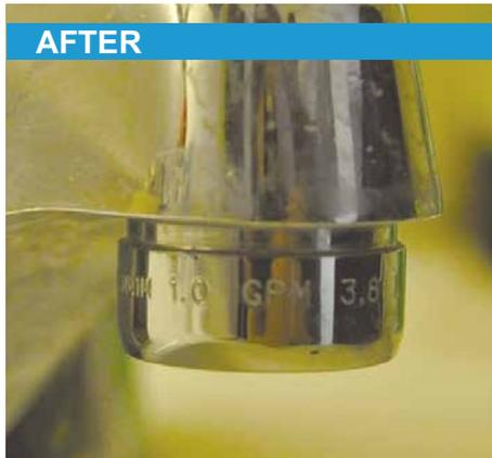
Low-flow faucet aerators limit flow to 2.2 gallons per minute or less and reduce water heating load by reducing water usage. [7.0201.1b.](#)
