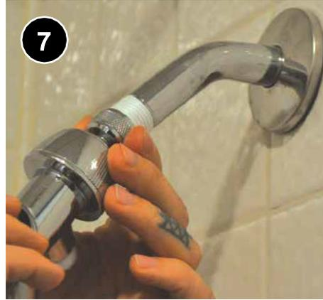
7 Install new showerhead according to occupant needs, such as handheld, shut-off, or swivel.
