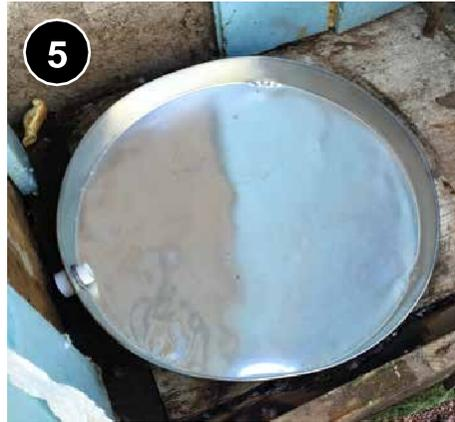
5 If the HPWH will be installed in or above conditioned space or in a location where water damage could occur, install a drain pan according to IRC requirements. Drain the pan to the exterior of the building. [7.0302.3g.](#)
