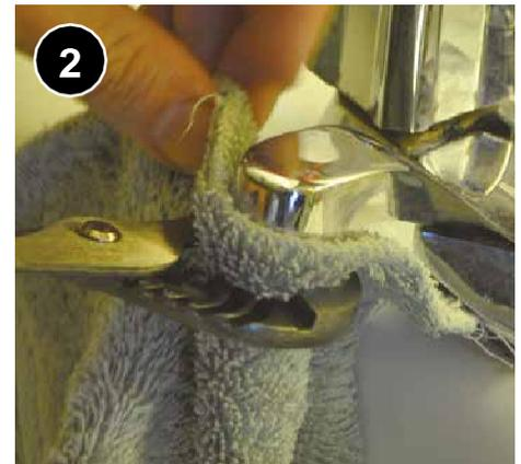
Using adjustable wrench or aerator wrench, gently remove old aerator, taking care not to damage faucet.
