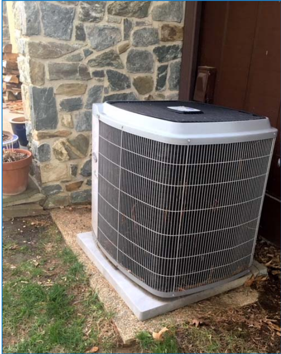
Heat Pump Slab Sloped Toward Corner
