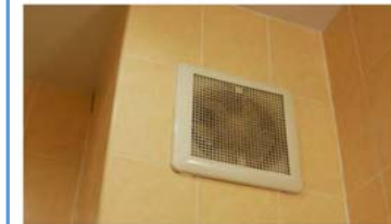
This bathroom exhaust fan is covered with dust so it may not be operating at full capacity.
