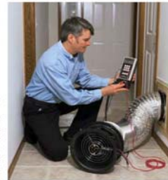
Duct leakage testing. A duct system can be tested for leakage using one of several methods to force air through the duct system under pressure and measure the air flow at different locations within the system. By comparing the pressures and flow rates, the test is able to determine the total amount of leakage and the location of any leaks in the system.
