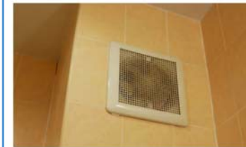
This bathroom exhaust fan is covered with dust so it may not be operating at full capacity.
